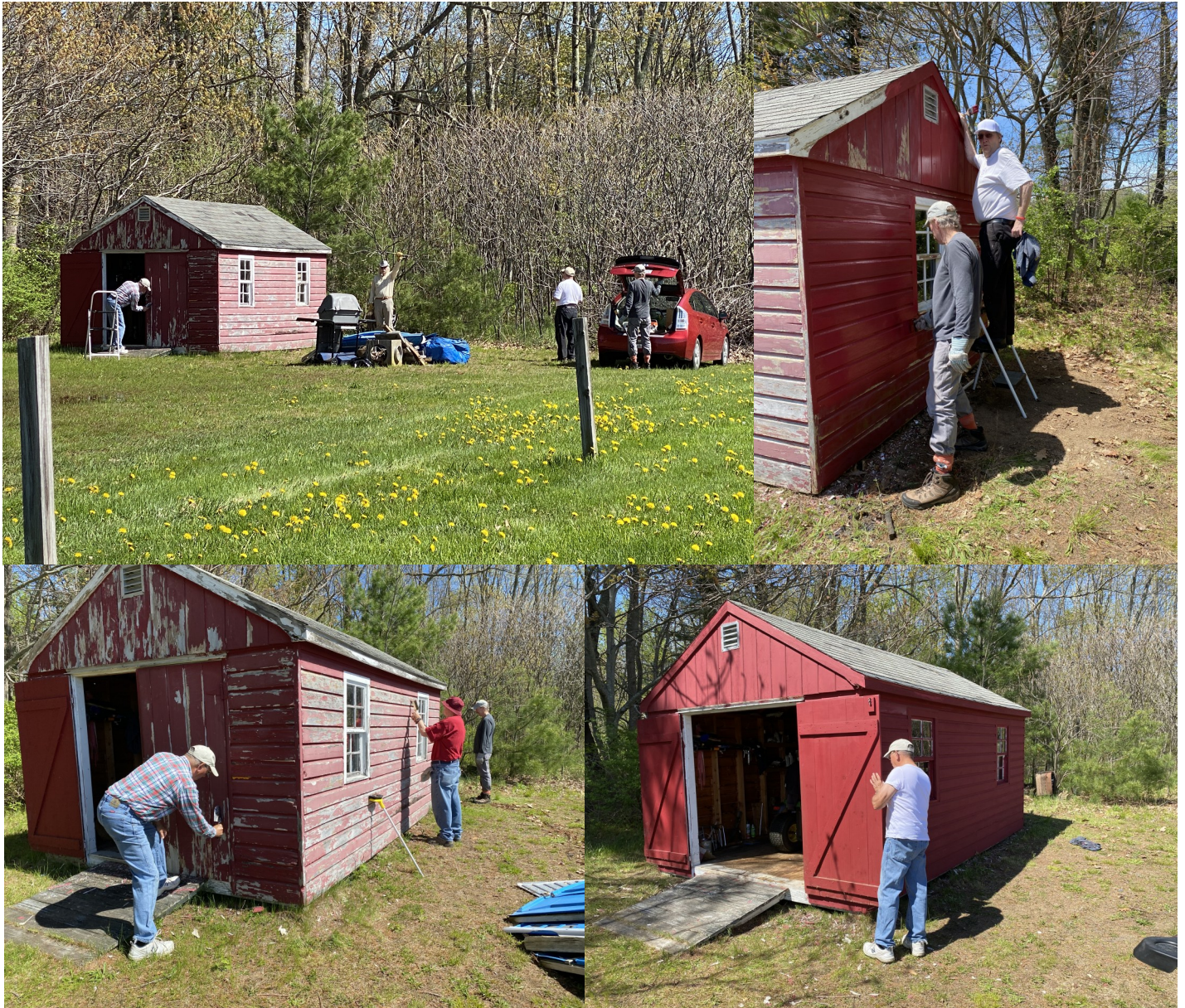
The shed got scraped and painted.
